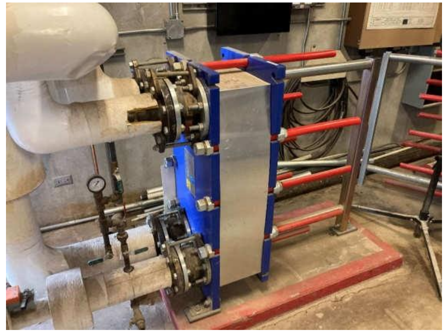
Basement Area – Geothermal Heat Exchanger
