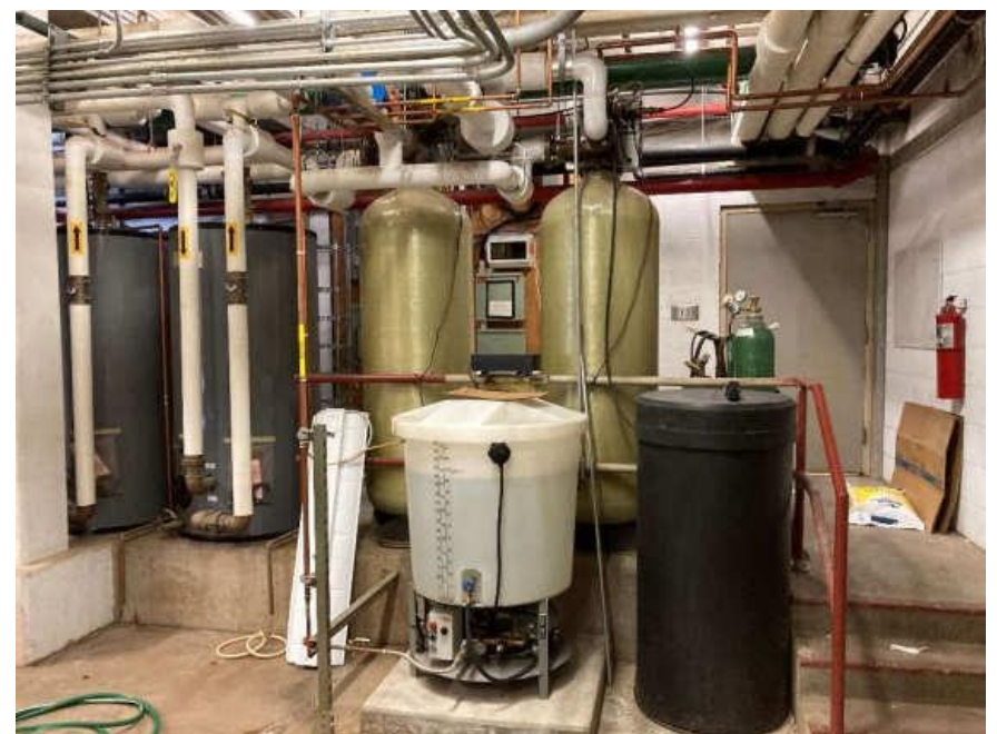
Basement Area – Water Softening System
