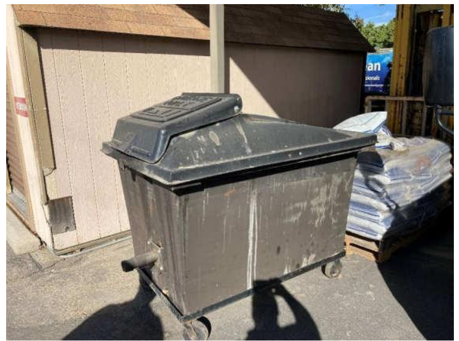
250-Gallon Portable Used Fryer Oil AST
