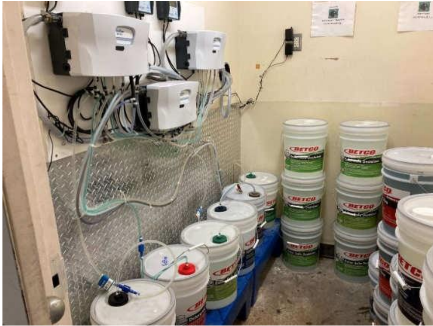
Laundry – Chemical Storage/Feed Pumps
