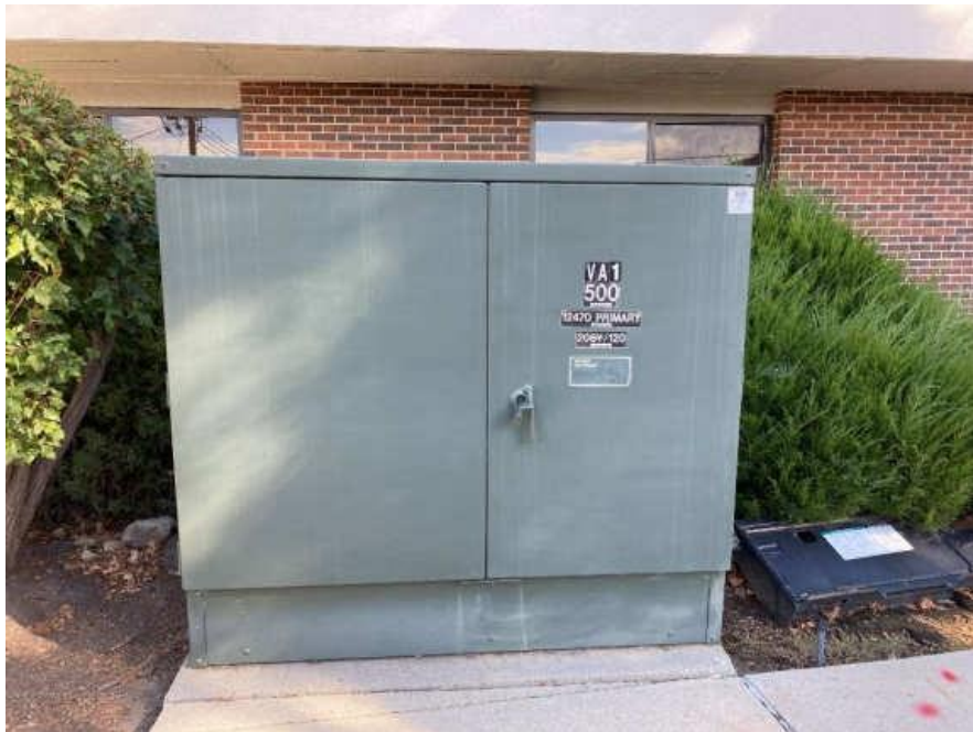
Pad Mounted Transformer
